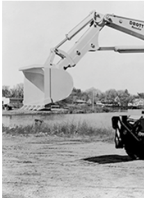
CASE enters excavator market.
